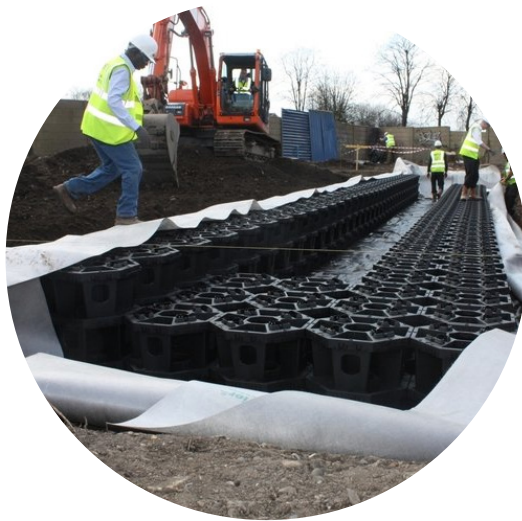
Example of structural soil cells
