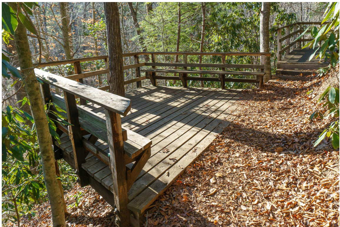
Viewing platform overlooking the Muskoka River
